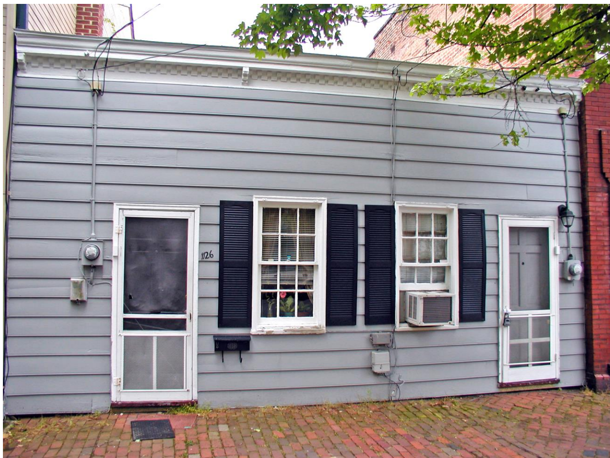
A building at 1126 Prince Street, said to have been an oyster house in the nineteenth century.
